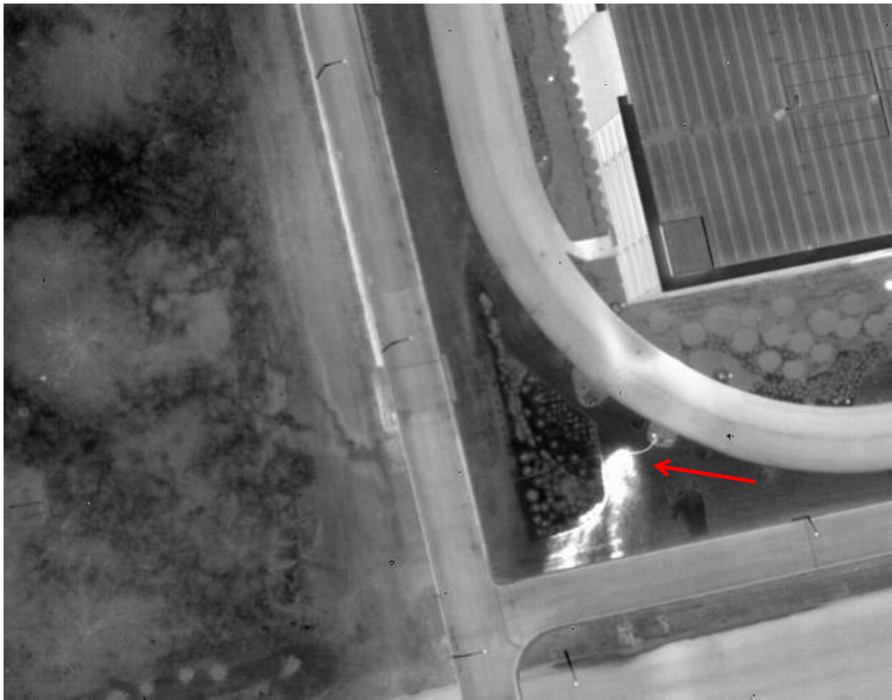
Figure 2) Steam line leaking onto the ground surface.
