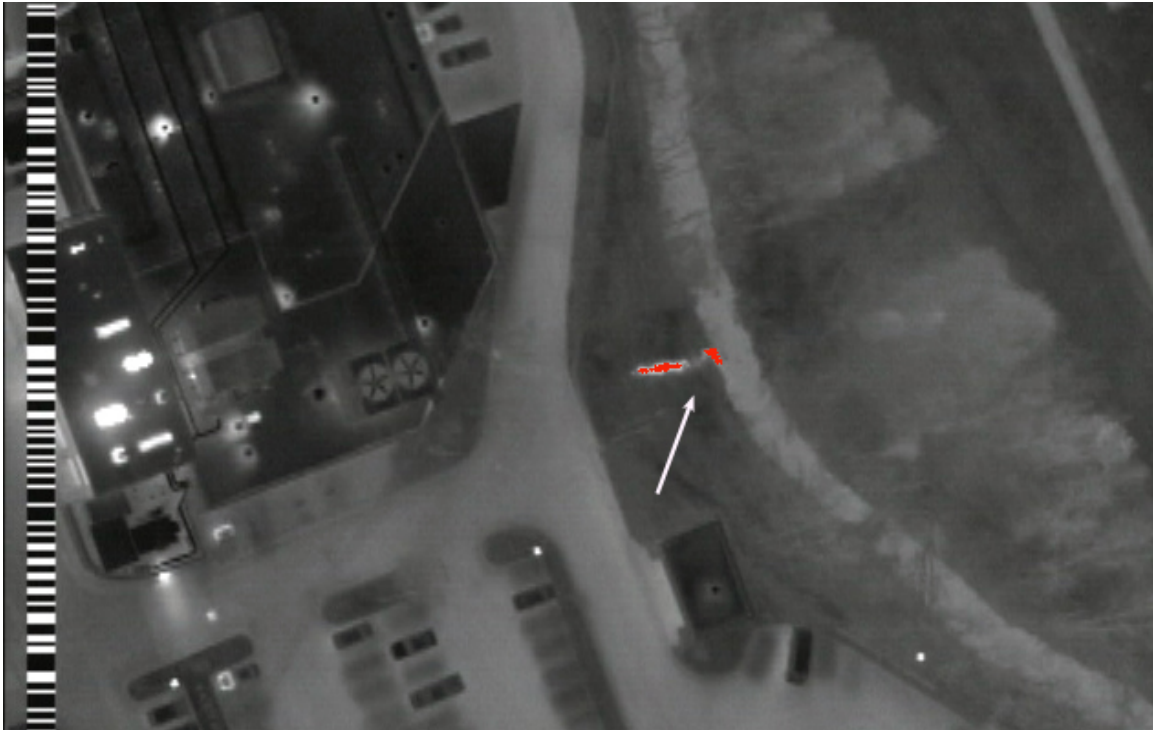
Figure 5) Thermograph of a storm drain (highlighted in red) leaking wastewater down to the bank of a creek and joining the flow. The leak is coming from the adjacent building.
