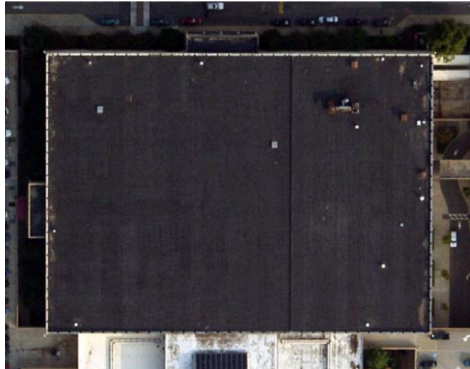
Figure 4b) Thermograph of a roof.
