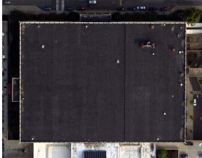
Figure 4b) Thermograph of a roof.
