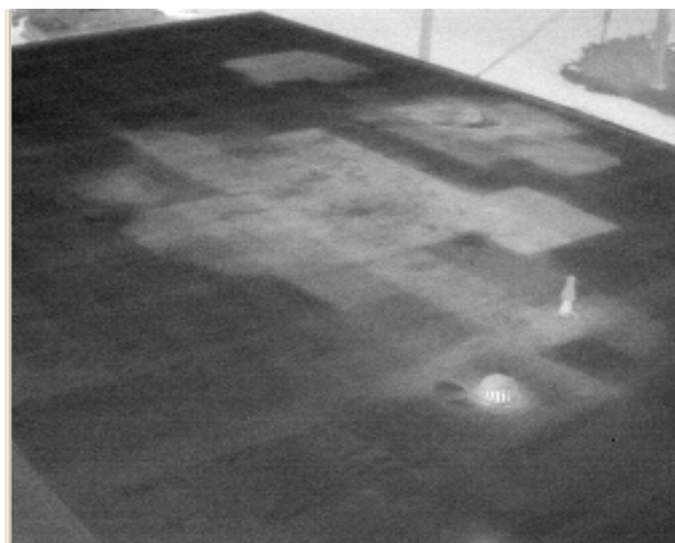
Figure 2) On-roof IR image.
