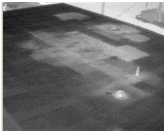
Figure 2) On-roof IR image.
